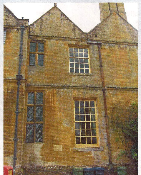
Stanway – the history of windows in one wall.
