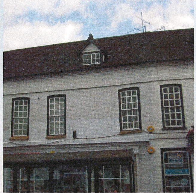
Early sash windows in Pershore are flush with the surrounding walls
